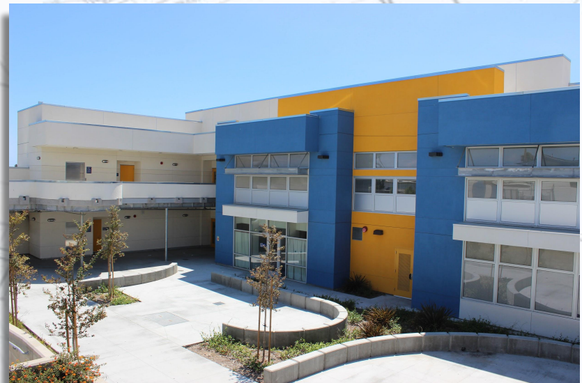
Knox Middle School: Before, During, After
